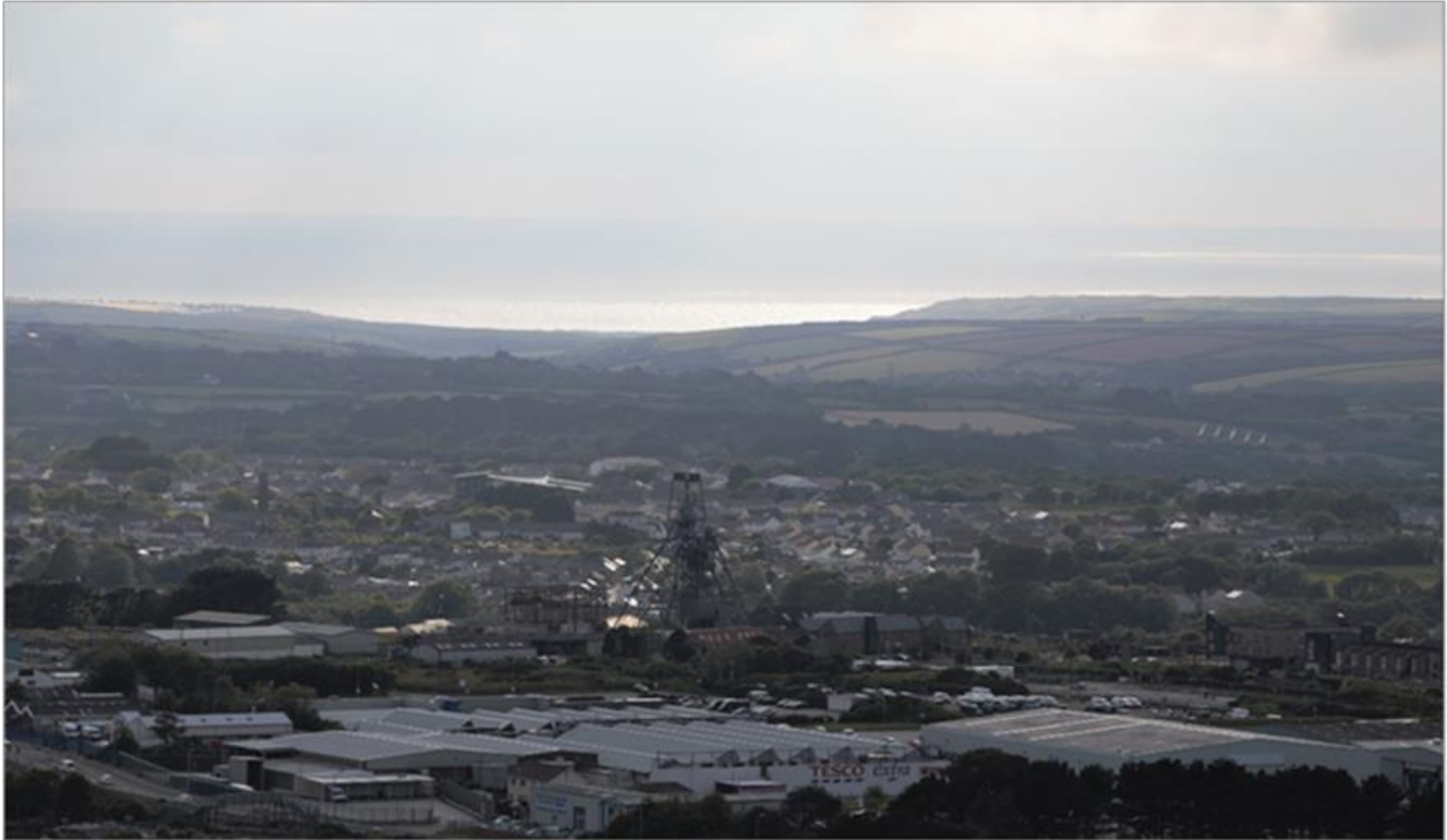
Figure 5.3 Photograph of the New Cook’s Kitchen headframe
